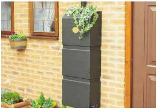
**Figure 113:** Example of a gravity fed rainwater system for flushing a downstairs toilet or for irrigation, elsewhere in the UK.
